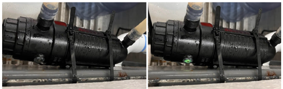
The difference between the UV lamp off (left) and UV lamp on (right) is subtle. It's important to check your system carefully and frequently.
